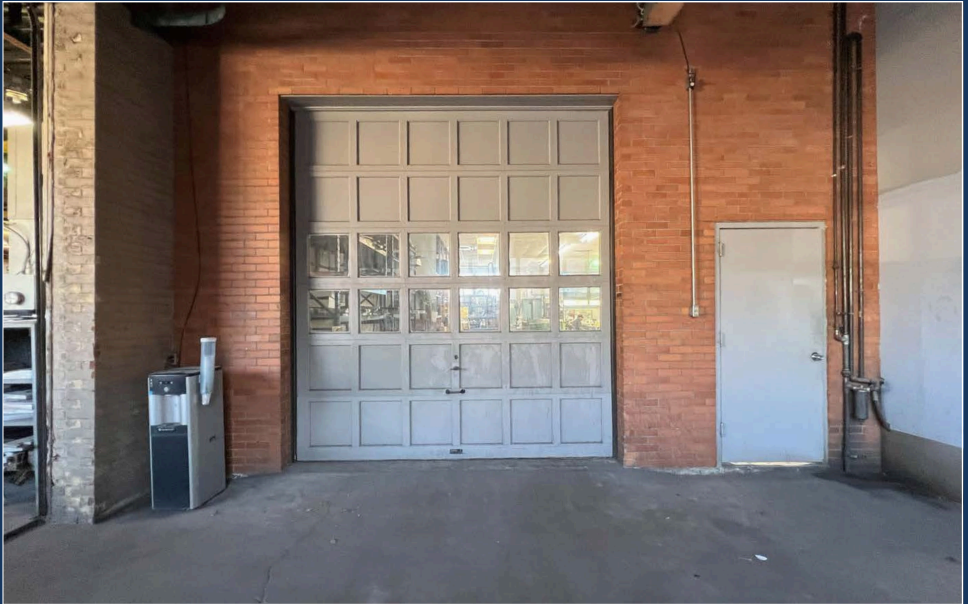
Two Interior Overhead Doors
