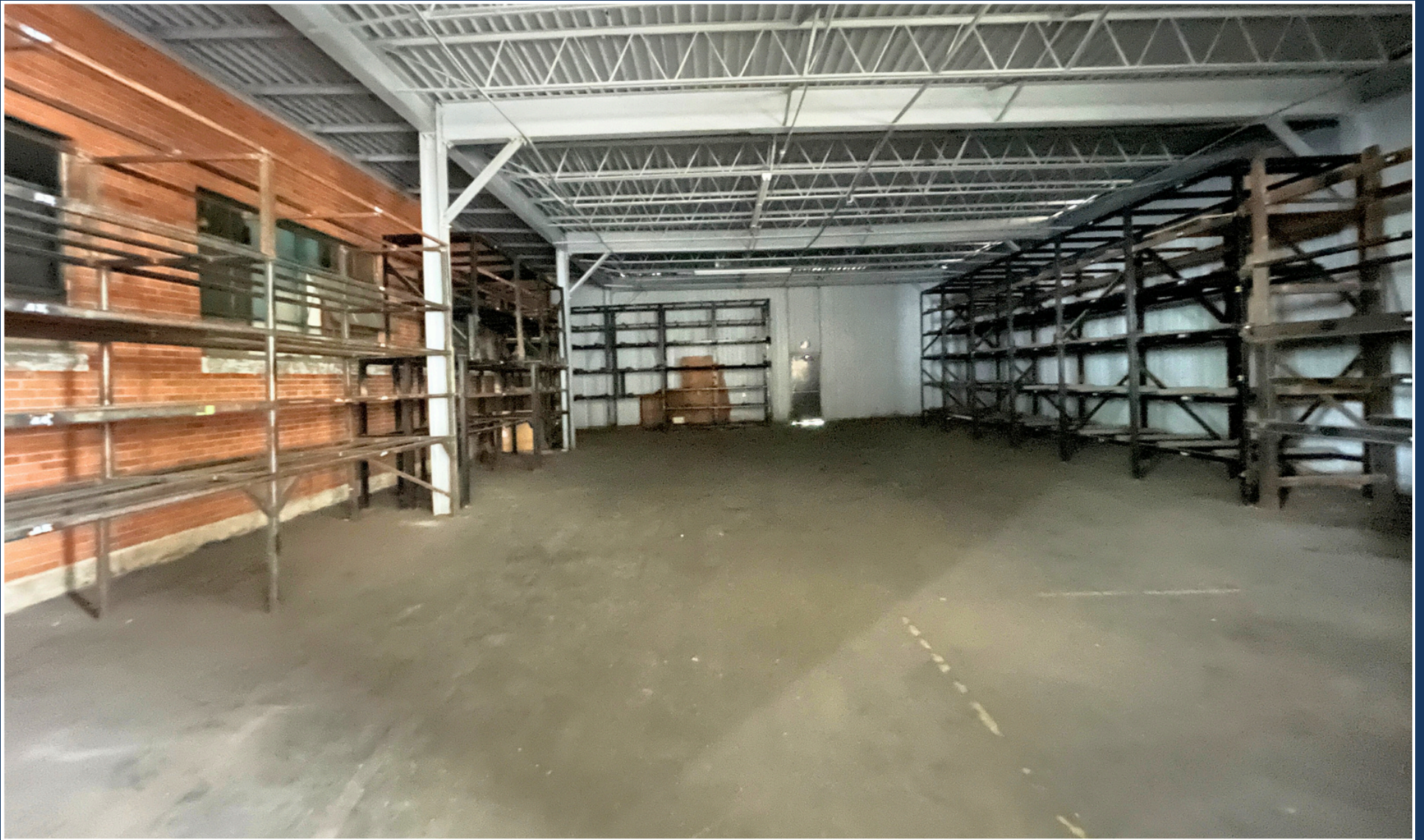
Interior Warehouse Room with Overhead Door
