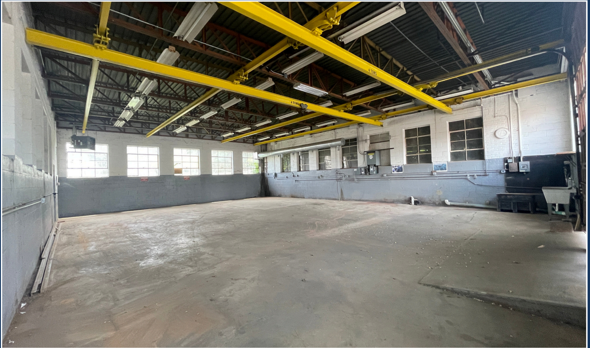
Warehouse Room with 4 Ton Overhead Bridge Cranes
